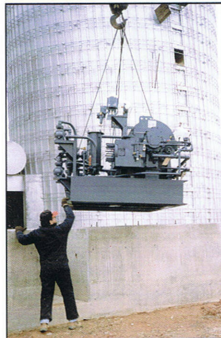
Turbine in flight toward its foundation
